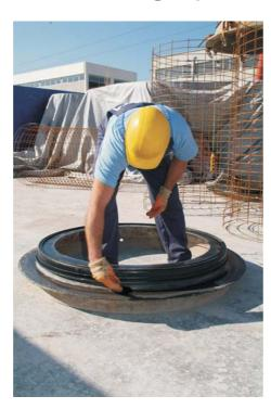
**SECIL** Integrated seal stretch on the cleaned and lightly oiled base ring. Ensure correct seating and even pre-stretching of the sealing ring.
